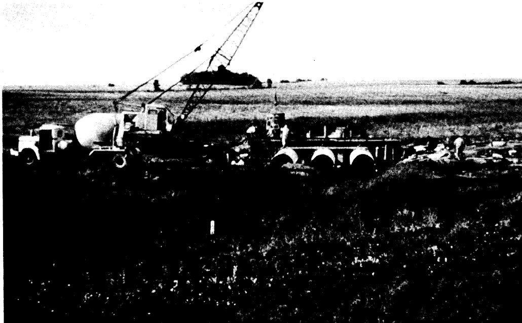
A water control structure being constructed in a wetland area.
