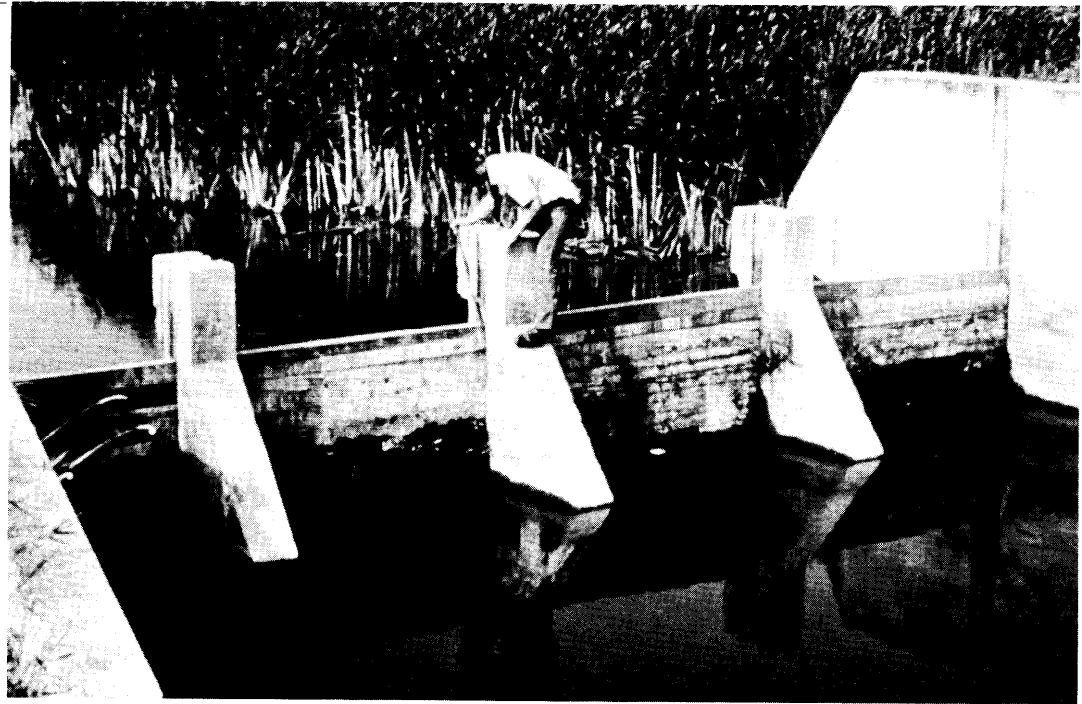
This structure controls water levels on the marsh to encourage growth of beneficial aquatic vegetation.
